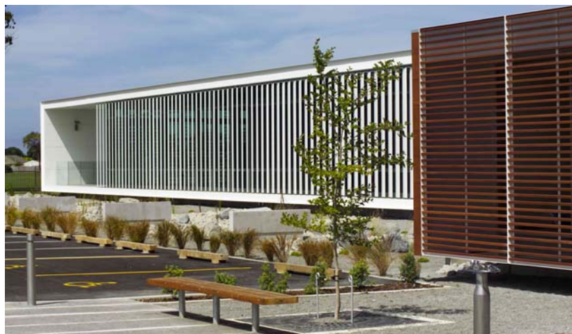
Main South Road view of library
